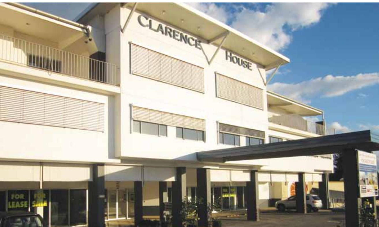
*Clarence House in Moss Vale, Sydney, was built using the Mi Panel technology; no brick work was included in the structure other than in the initial foundation.*
